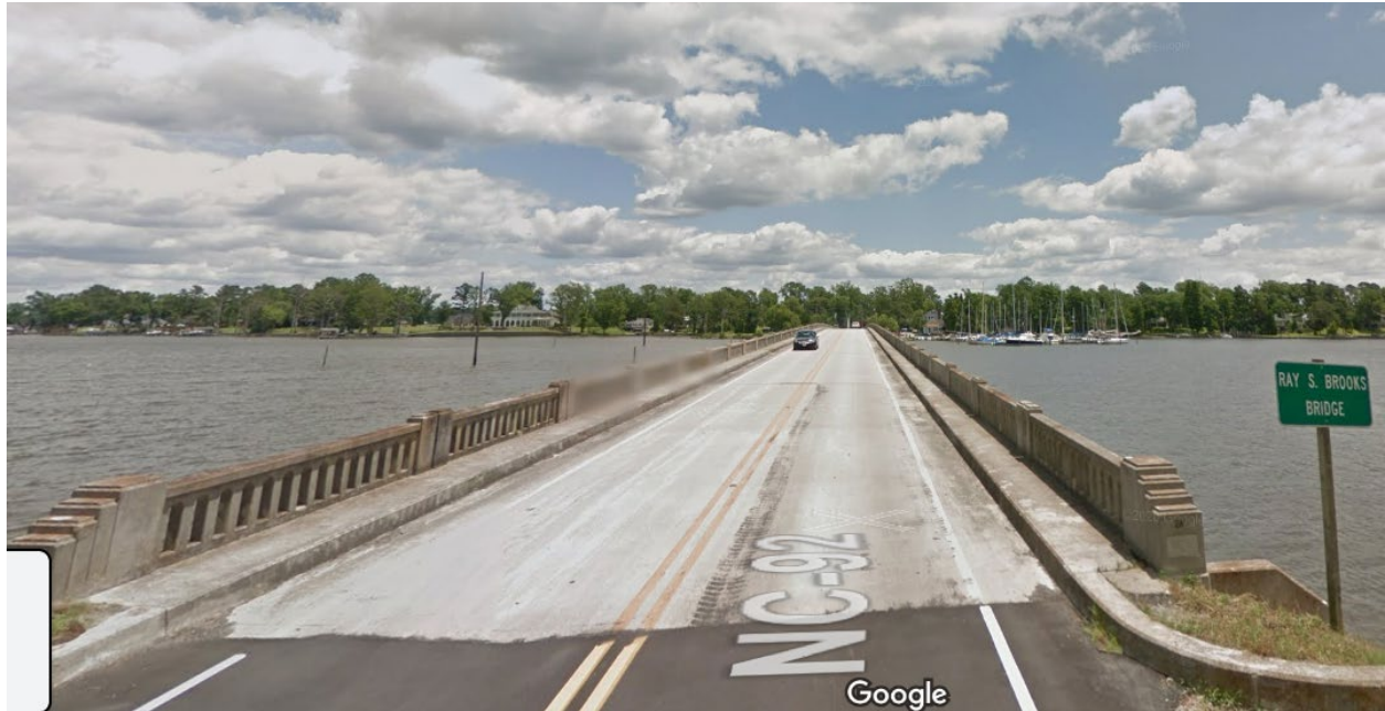
NC-92 bridge over Bath Creek
