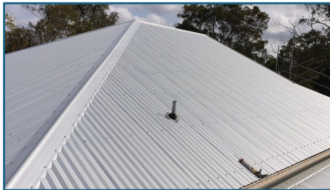
5V Tin Roofing
