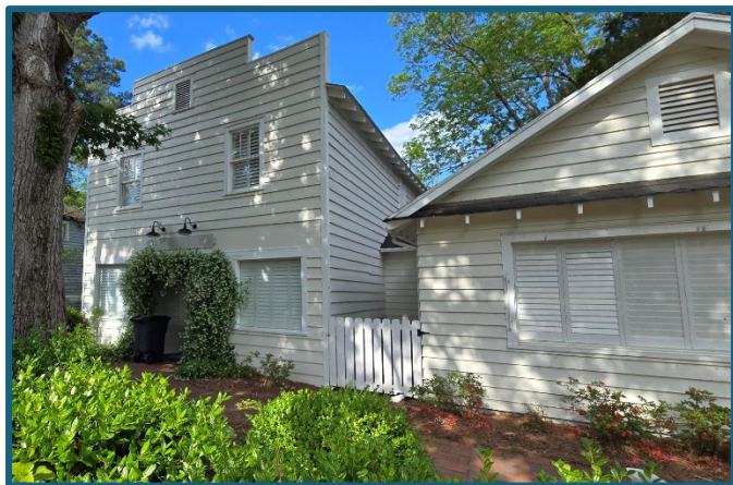
Wood Siding – Properly Preserved
